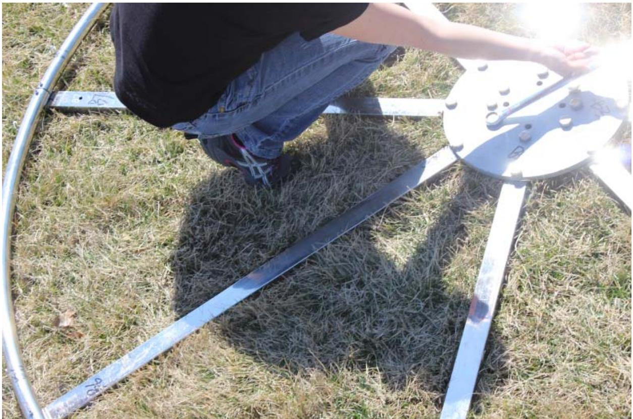
Attach the telescopic pole to the bottom plate.
