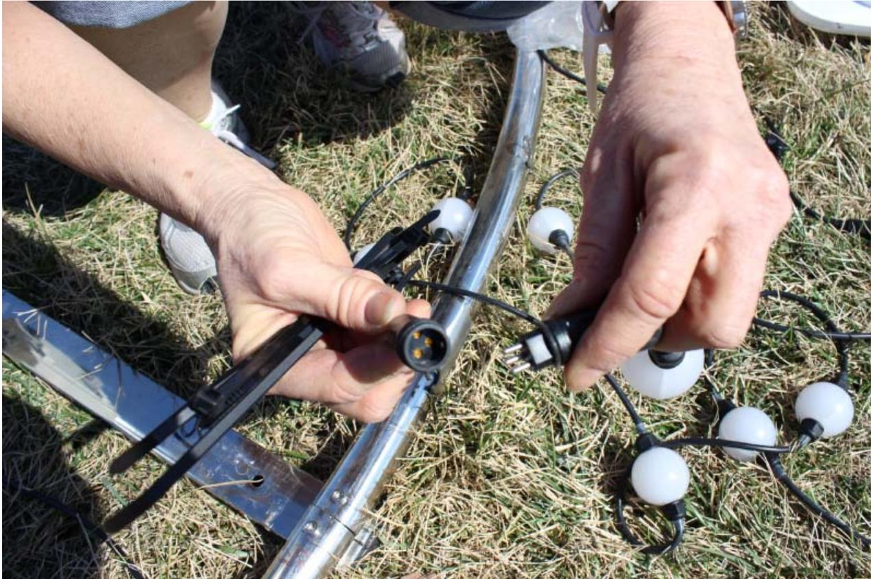
Take the center of the two strings (where you joined them together) and cable tie it to the nearest loop on the top ring. Each pair of strings should take up the space of two loops.
