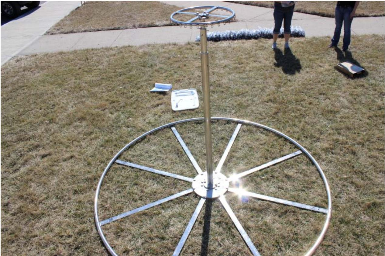
Attach your light controller to the telescopic pole. Be sure to mount the controller at least 2 ft from the ground to minimize the potential for water to enter the enclosure.
