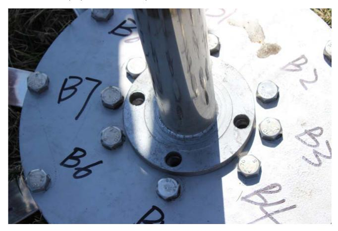
Put the lockwasher in place, then insert the bolt for all four hole on the telescopic pole.
