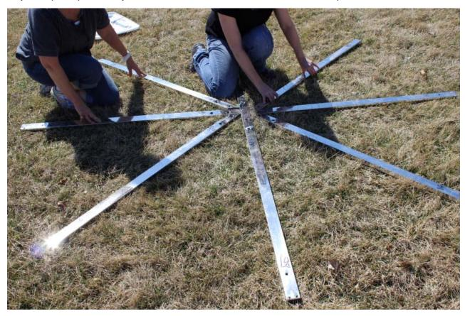
Match the bottom plate numbers to the numbers on the spokes and bolt the plate onto the spokes, but do not tighten bolts.
