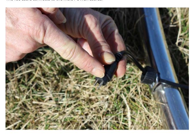
Connect the male POWER cable with the female at the "bottom" of the Tee and tighten the connection.
