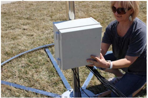
Your controller will have 4 cables coming from it that are labeled 1, 3, 5 and 7. These are the DATA cables. These will correspond to the labels on the spokes of the lower ring. So, cable 1 will be placed near the edge of the ring on spoke B1. Cable 3 will be placed near the edge of the ring on spoke B3 and so on.
