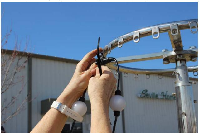
Now connect the female connector on the two strings to the male end of the Tee connector nearest to the data connector labeled "1".
