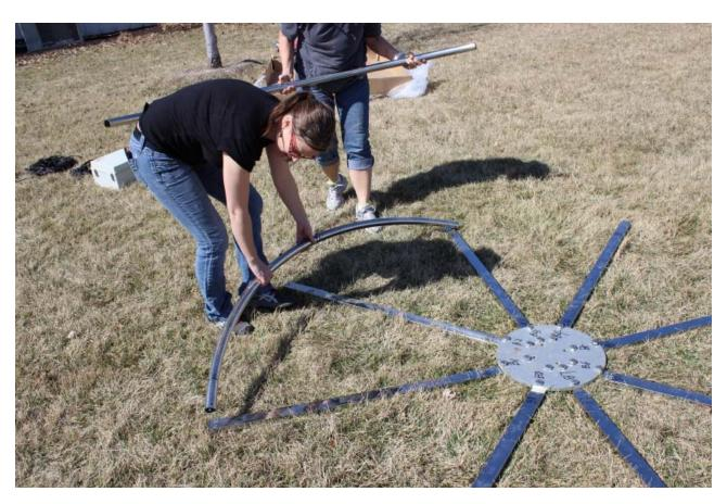
Match the labels and join the ring pieces with the spoke pieces using the Allen screws.
